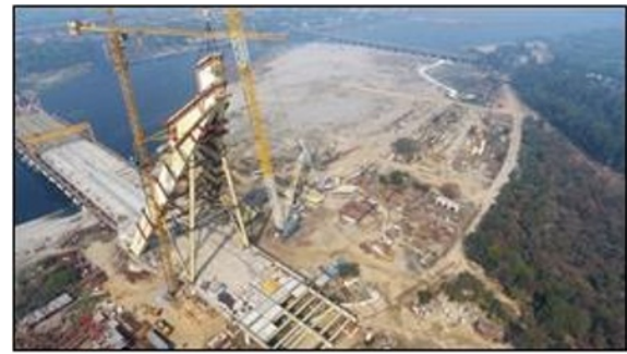
Fig. 6. Construction of Signature bridge.
