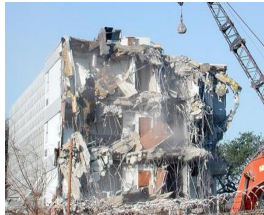
Fig. 2. Dismantling of Building.
