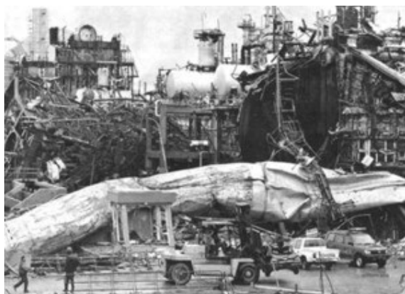
Fig. 3. Skikda, Algeria, January 19, 2004: LNG Plant explosion due to liquid metal embrittlement [10].
