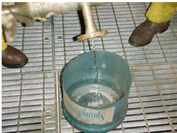
Fig. 2. Liquid mercury removal during gas equipment maintenance. Courtesy of Petronas.
