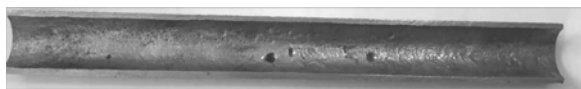
Fig. 7. The nature of damage to the inner surface of the tube after Stripping from deposits.
