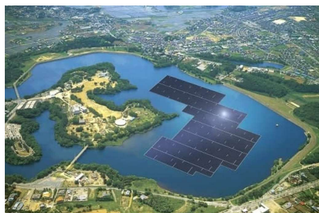
Fig. 1. A floating photovoltaic plant at the Yamakura Dam in Ichihara
