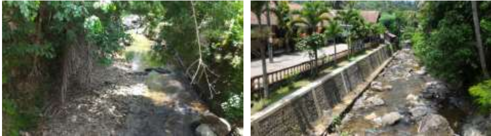
Fig. 9. Deposition on river bed at Loc.1.
