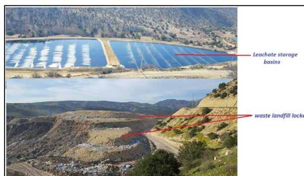
Fig.1. Panoramic view of Landfill of Tamelast (Source: Field survey, 2017).
