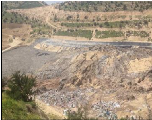
Fig.13. Slide of a damaged household waste landfill locker (Source: Field survey, 2017).
