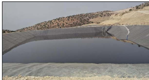
Fig.22. Geomembrane of the leachate storage basin at the Tamelast landfill site.
