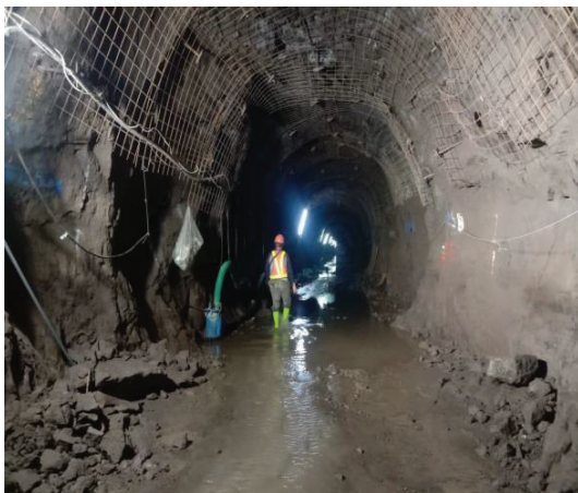
Fig. 11. Rock bolt, wire mesh, and shotcrete installations.
