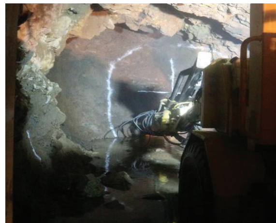
Fig. 9a. Tunnel excavation: Drilling.
