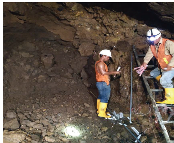
Fig. 9b. Tunnel excavation: Charging.
