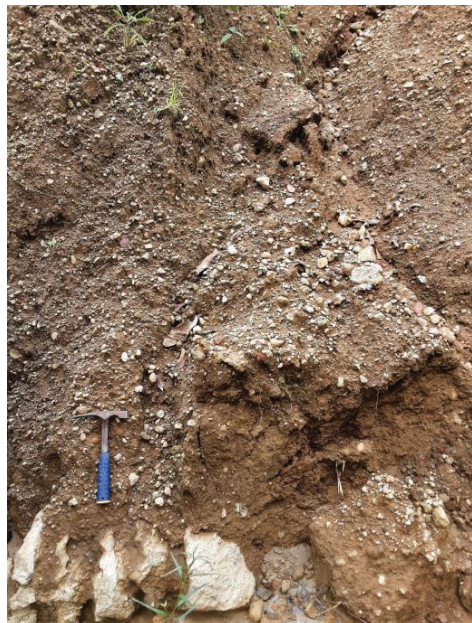
Fig. 6. Highly weathered andesitic breccia in ST 5.
