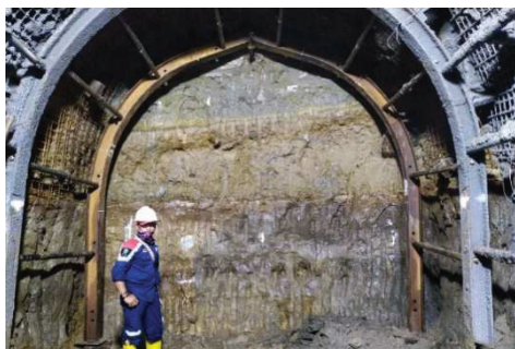
Fig. 5. Appearance of lapilli tuff on the outlet tunnel face
