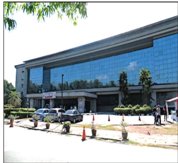
Fig.2. Front part of UNITEN administration building.
