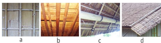
Fig. 8. Bamboo material for (a) wall, (b) ceiling, (c) roof frame, and (d) roof of sago leaf.
