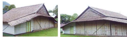
Fig. 6. The roof of Folajiku Traditional House.
