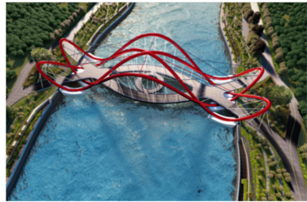
Fig3. Effect picture of flying-swallow style cable-stayed arch bridge with Lissajous curve arch rib
