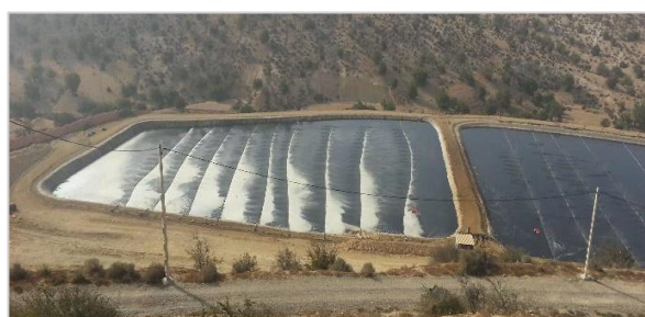
Fig. 4. Saturation of leachate storage ponds up to 6 ponds
