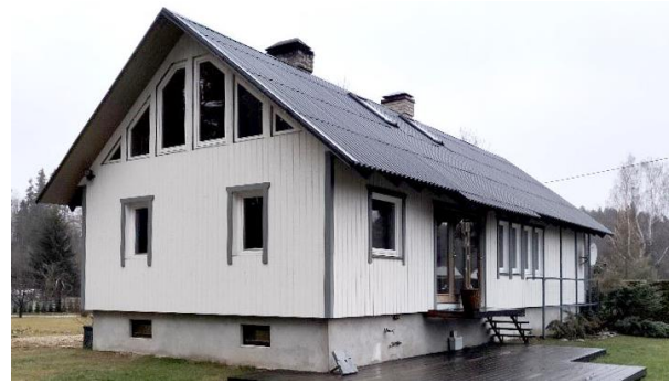
Figure 1. View from west of the single-family building before renovation.
