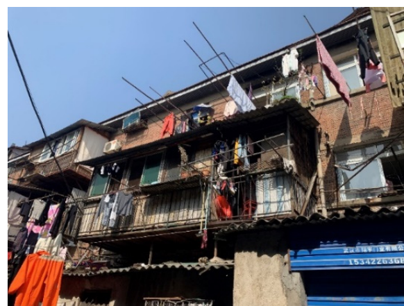
Fig. 3. Houses build by the residents themselves
