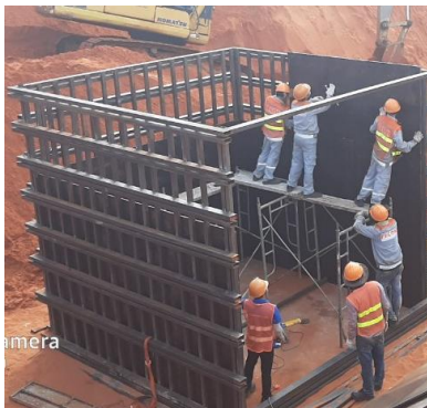
Fig. 4. Setup formwork for mockup with styrofoam 5cm.
