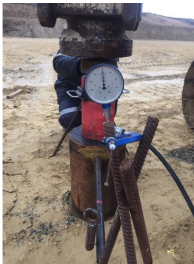
Fig. 9. Die tests for determining the deformation modulus of a vibro stone columns
