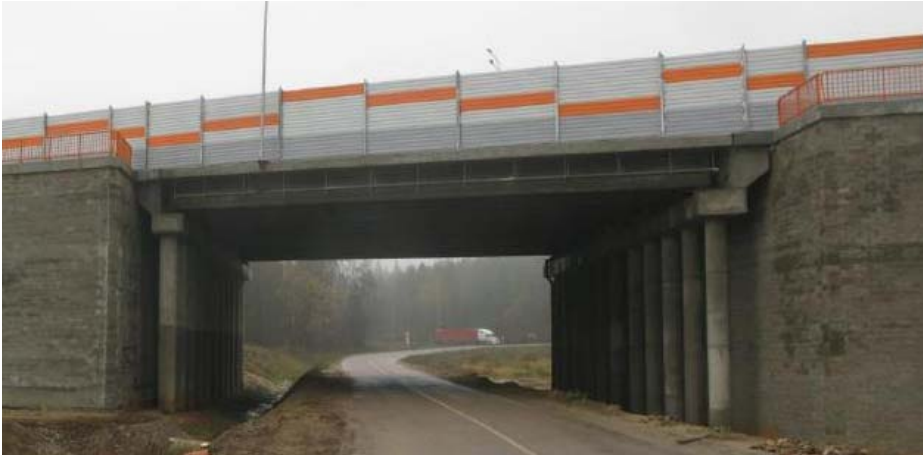
Fig. 10. Implemented version of the MSE-wall
