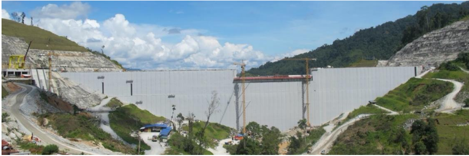
Fig. 2. SIBELON CNT exposed geocomposite system installed at Susu low cement content concrete dam, Malaysia, 2016
