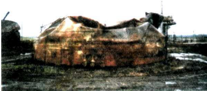
Fig. 1. The tank "collapsed" as a result of an explosion and fire.
