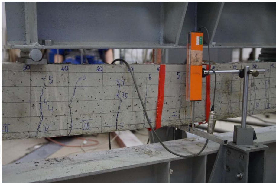
Fig. 3. Crack formation in beam reinforced with BFPR B2.6.3 at load P = 0,2 P_{ult}
