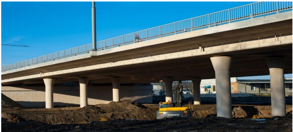
Fig. 1. The bridge is a continuous girder system.
