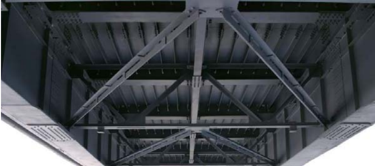
Fig. 1. Superstructure with orthotropic plate.
