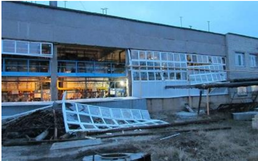
Fig. 1. Separation of bindings from window spans
