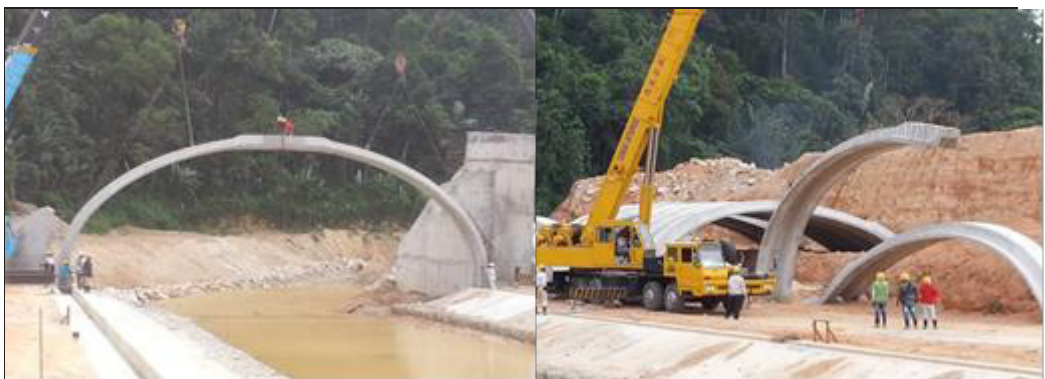
Fig. 2. Construction of backfill arched Road Bridge
