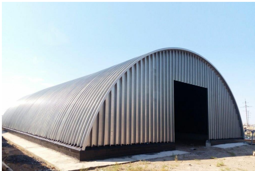
Fig. 1. General view of a frameless arched construction
