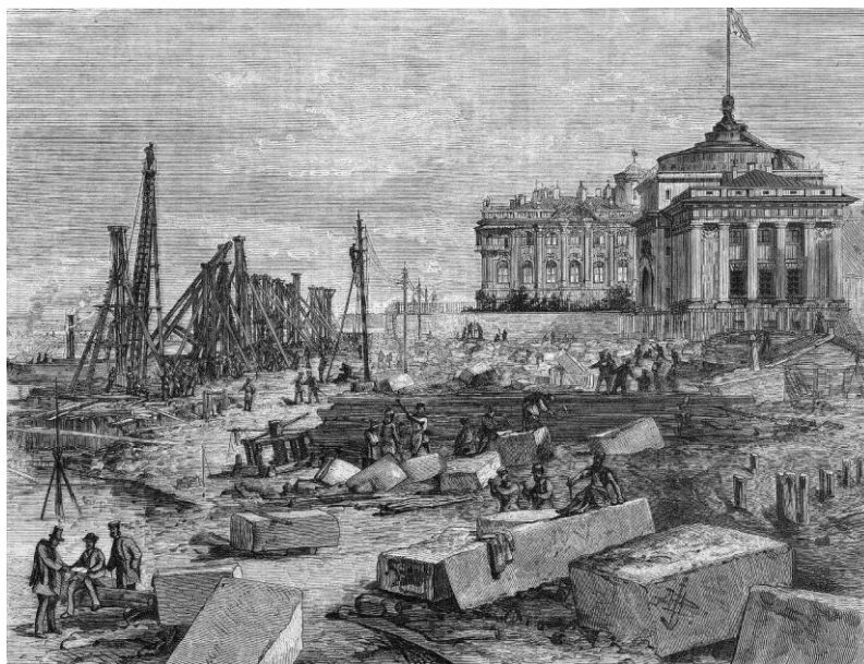
Fig. 4. Engraving. Construction of the Admiralty embankment (Beggrov, engraved Kammuller 1873).
