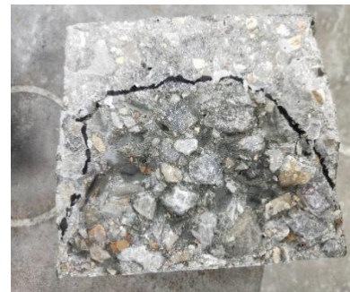
Figure 2. Depth of water penetration
