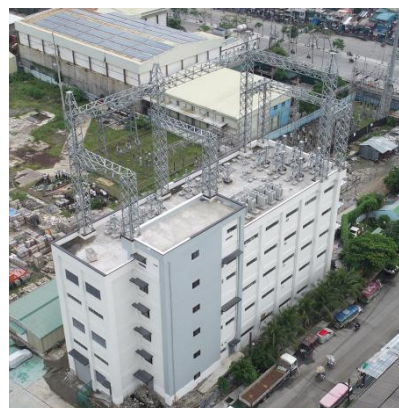
Figure 1. substation building in the Philippines
