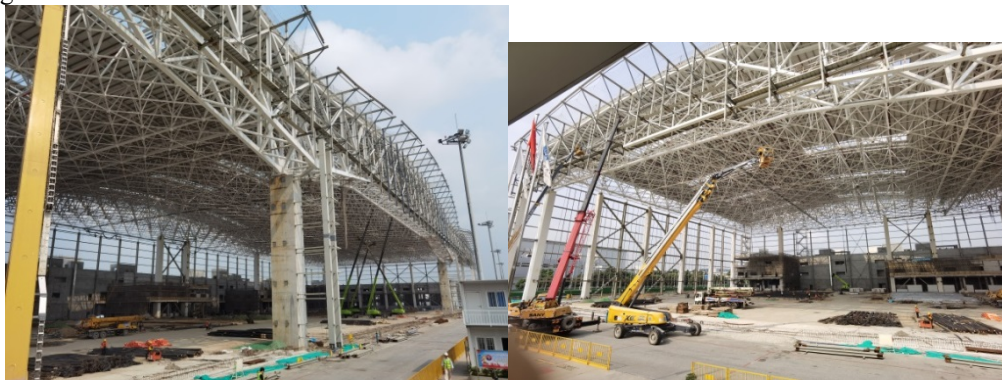
Figure 2. The third phase of GAMECO aircraft maintenance facility.
