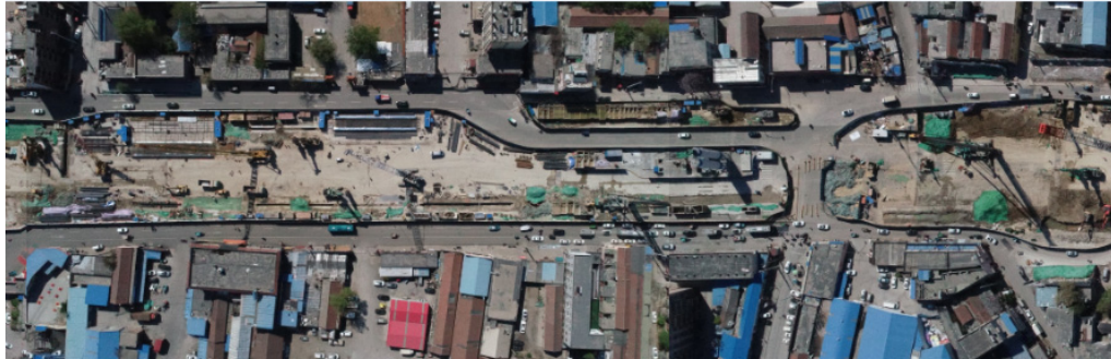
Figure 1. Aerial view of construction area.
