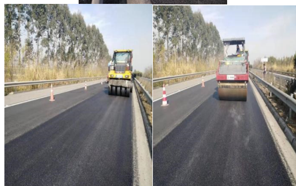
Figure 3 Combined Steel-Rubber-Steel Rolling Compaction Process
