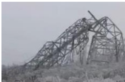
Fig.1. Collapse of power transition line, caused by icing
