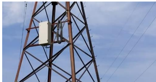
Fig. 2. Installing a smart-system on an overhead power line support
