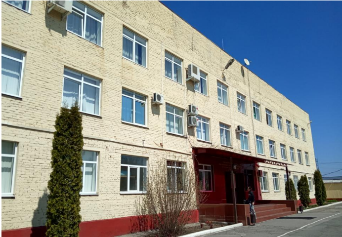
Fig. 1. General view of the reconstructed building
