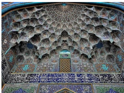
Fig. 14. Mosaic cladding in Sheikh Lutfalla Mosque, Isfahan, (Iran).
