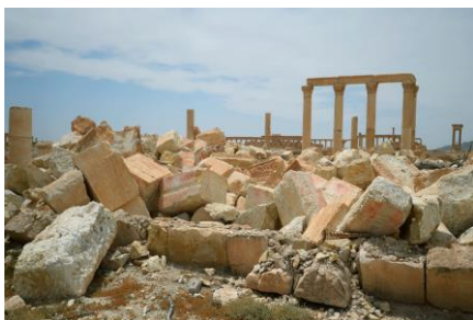
Fig. 5. Destroyed temples in Palmyra (Syria).
