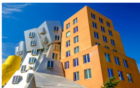
Fig. 14. Ray and Maria Stata Center (architect Frank Gehry).
