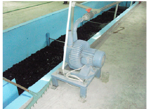
Fig.3 Aeration system of the biological filter
