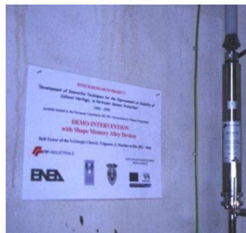
Figure 1. (c)Damper after installation
