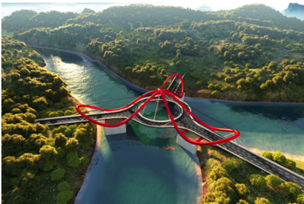
Figure 3. Three fork flying swallow cable stayed arch bridge
