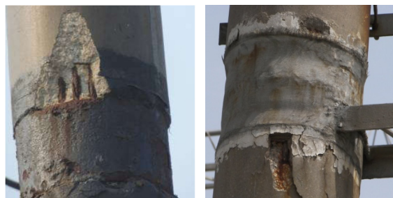
Figure 4. Triple corrosion coupling
