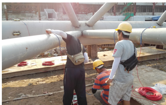
Figure 6. Installation of arch vault strain gauge
