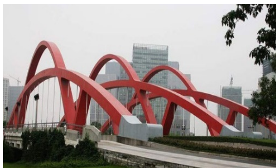
(a) Yuanshi Bridge
