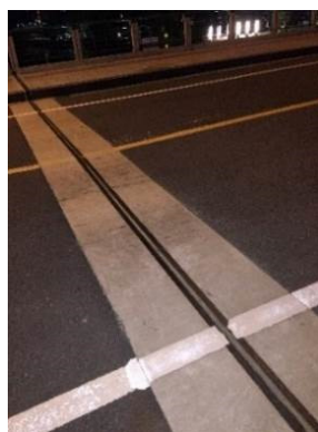
(a) Single-gap expansion joint (Cailian Bridge)
