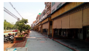
Figure 7. space outside pedestrian street
