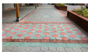
Figure 9. Floor paving with hexagonal brick
