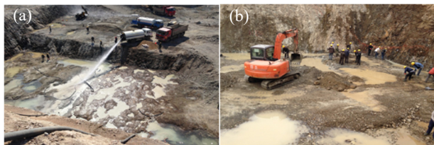
Fig. 4 Test site cleaning.
