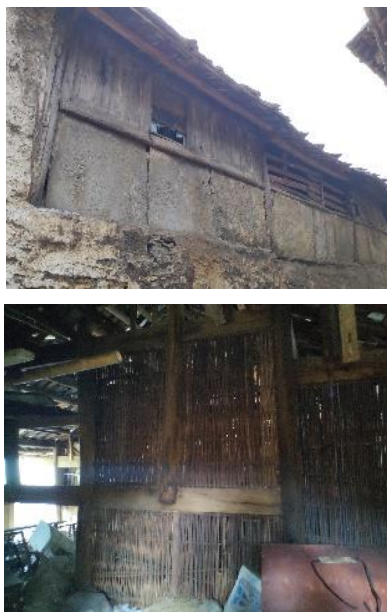
Figure 2-2-2 Types of non-load bearing walls Source: Author's own photos
