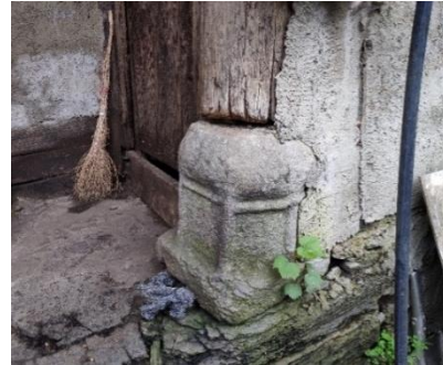
Figure 2-1-1 Column foundation appears Source: Author's own photos
