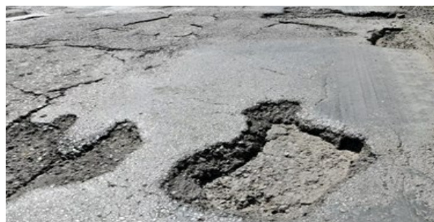
Fig. 3. Potholes
