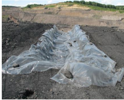
Fig. 2. Waterproofing of the bottom and slopes of the WWTF ditch
