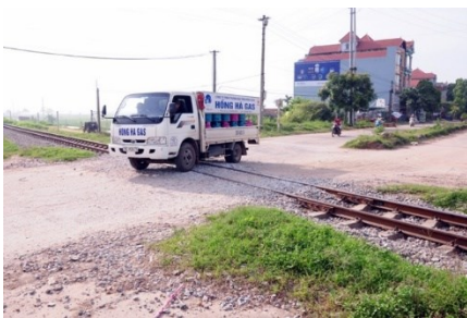
Fig. 8. The intersection has no barrier [13]
