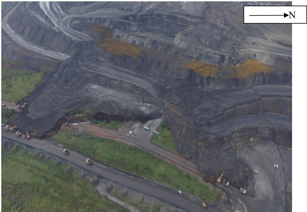
Fig. 3. Landslide of the External dump at the mine ‘R’ (photo from a quad-copter)
