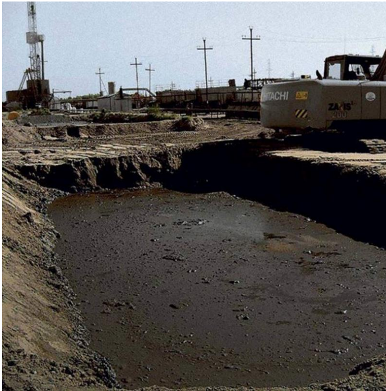
Fig. 1. Waste pit on the drill site.
